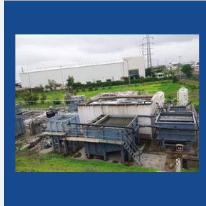
Sewage Treatment Plant
